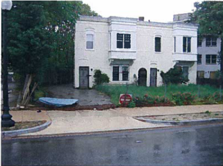
1414 Maryland Avenue – Longstanding Vacant Property
