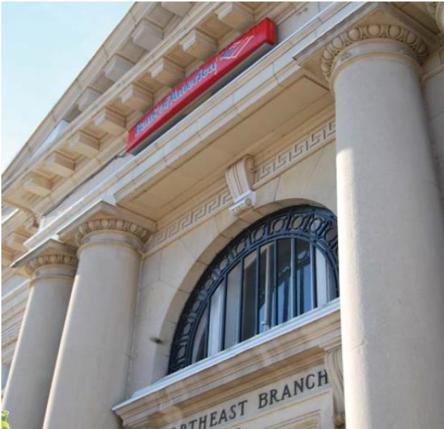
"Northeast Branch" signage is historic example of lettering applied to fascia. However, the "Bank of America" signage appears incongruous to the classical, architectural facade elements. Also, concealment of electrical conduit is preferred.
