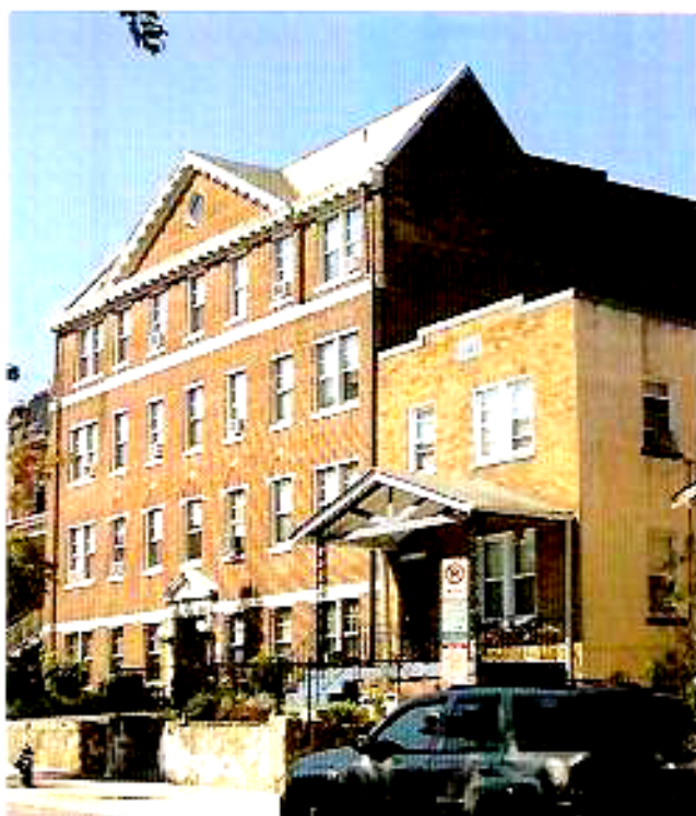
Existing 4 story 13th Street between F and Emerald
