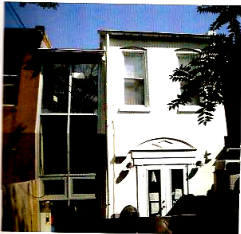
Rear Facade of (Subject House)
