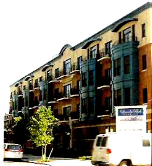
New 4 story 13th Street between Emerald and
