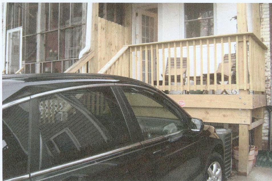
Existing back deck
