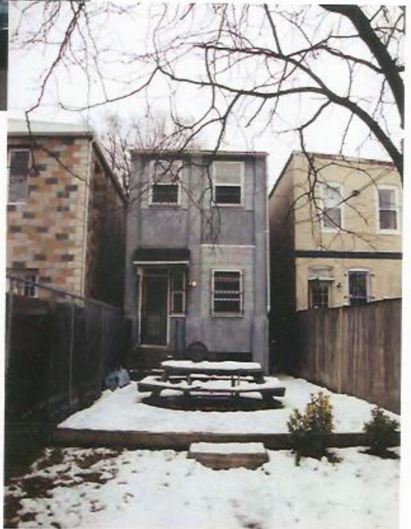
Rear of 808 9th Street NE
