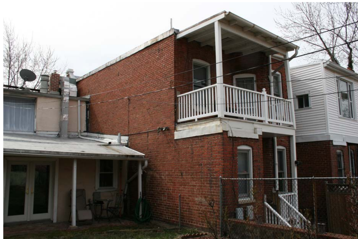
View of rear towards Southwest
