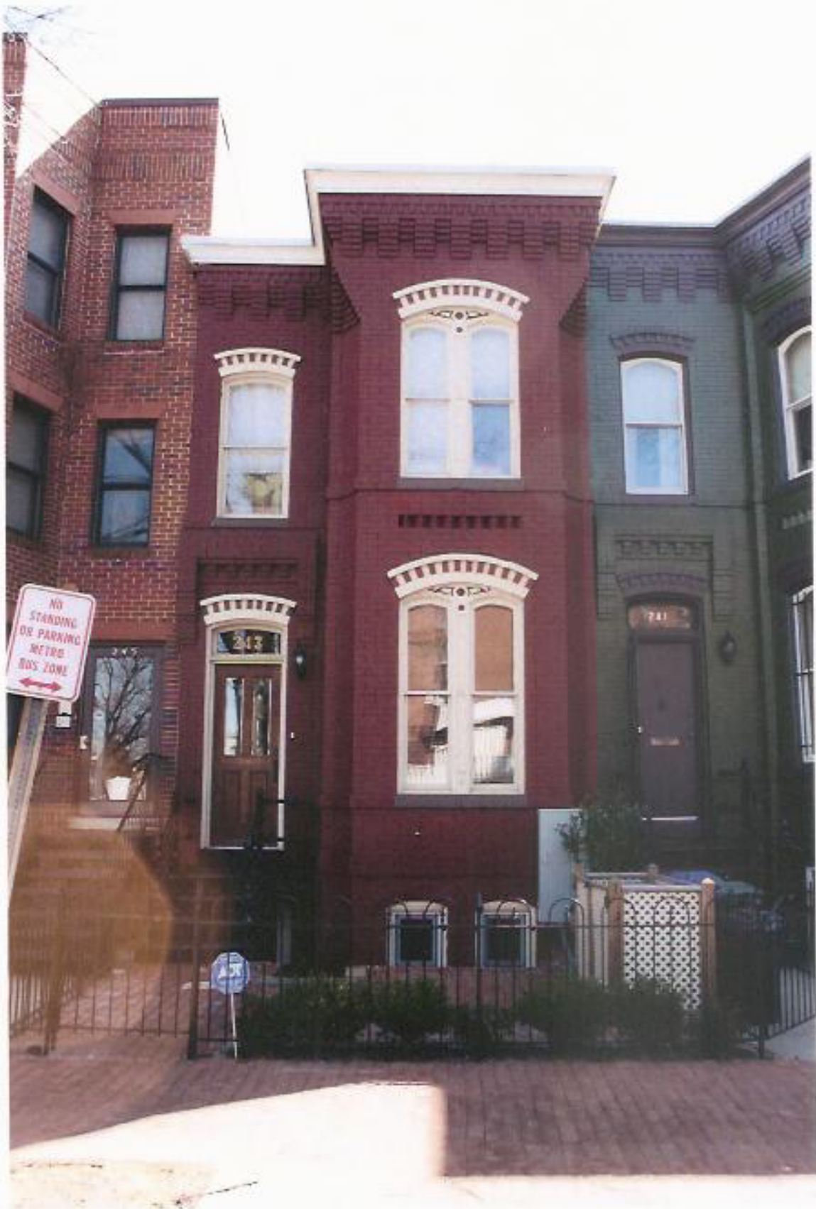
Street Frontage 243 8 th Street NE
