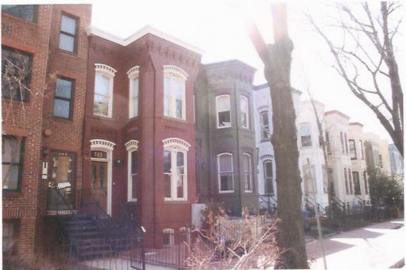
View from 8 th Street NE towards South
