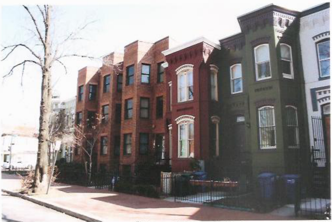
View from 8 th Street NE towards North
