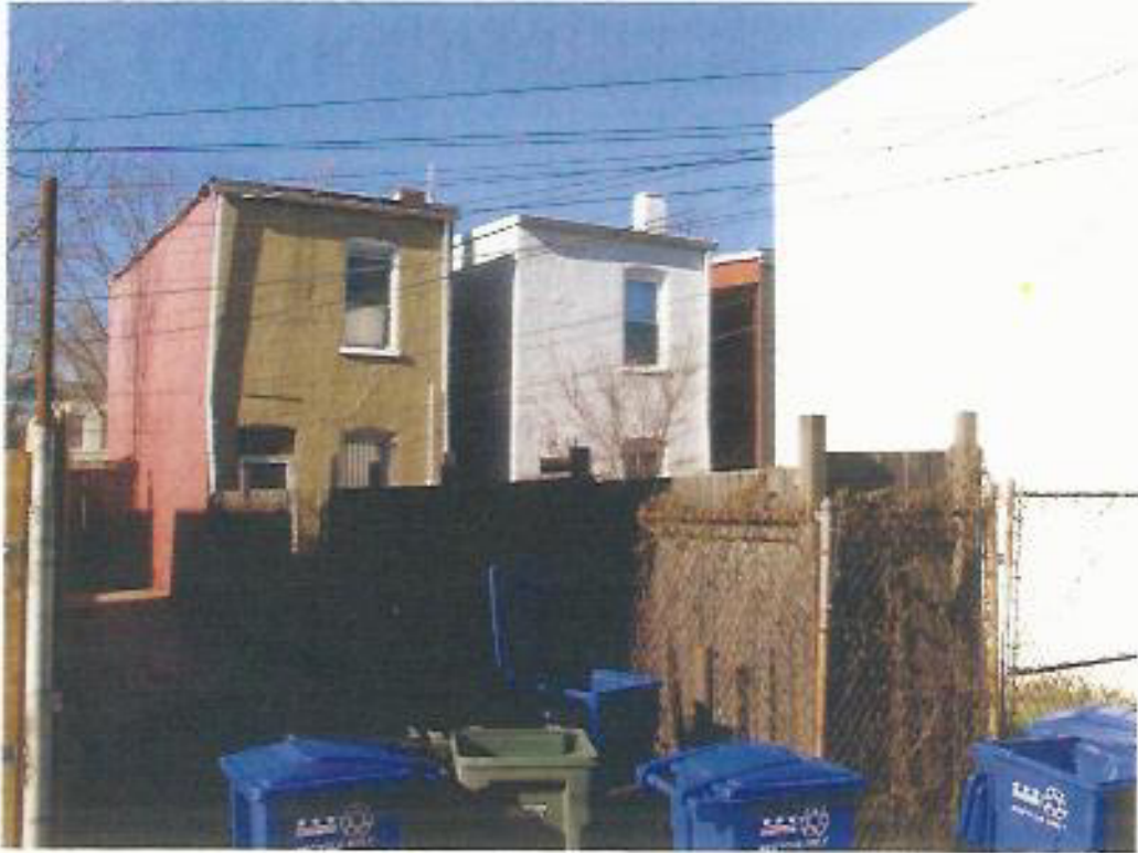
VIEW TO THE NORTH
