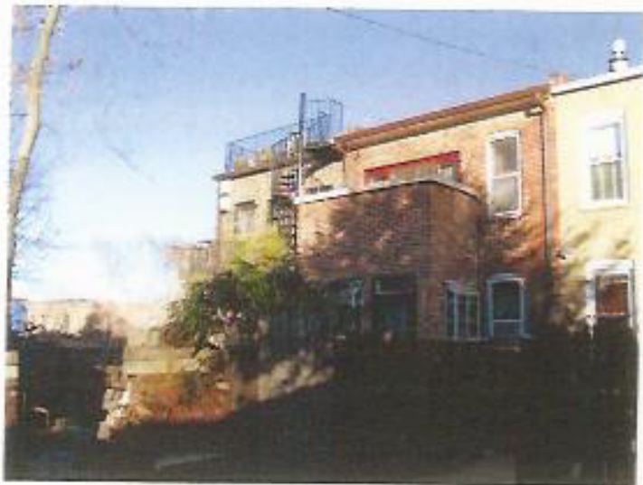
VIEW TO THE NORTH
