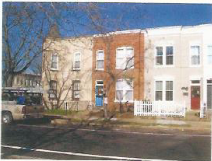
VIEW TOWARDS 14 TH STREET
