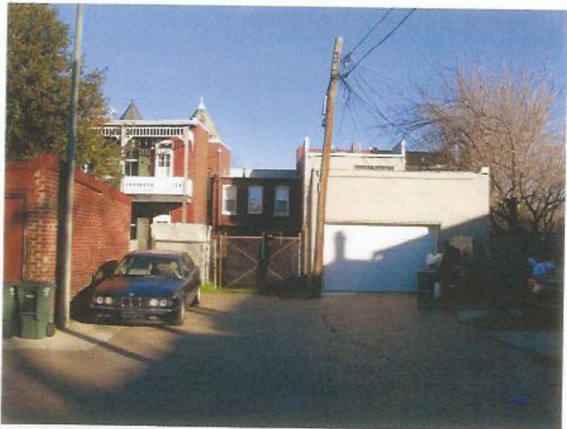
DEAD END ALLEY TO THE SOUTH
