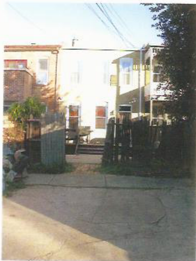
REAR VIEW OF 312 12 th STREET NE
