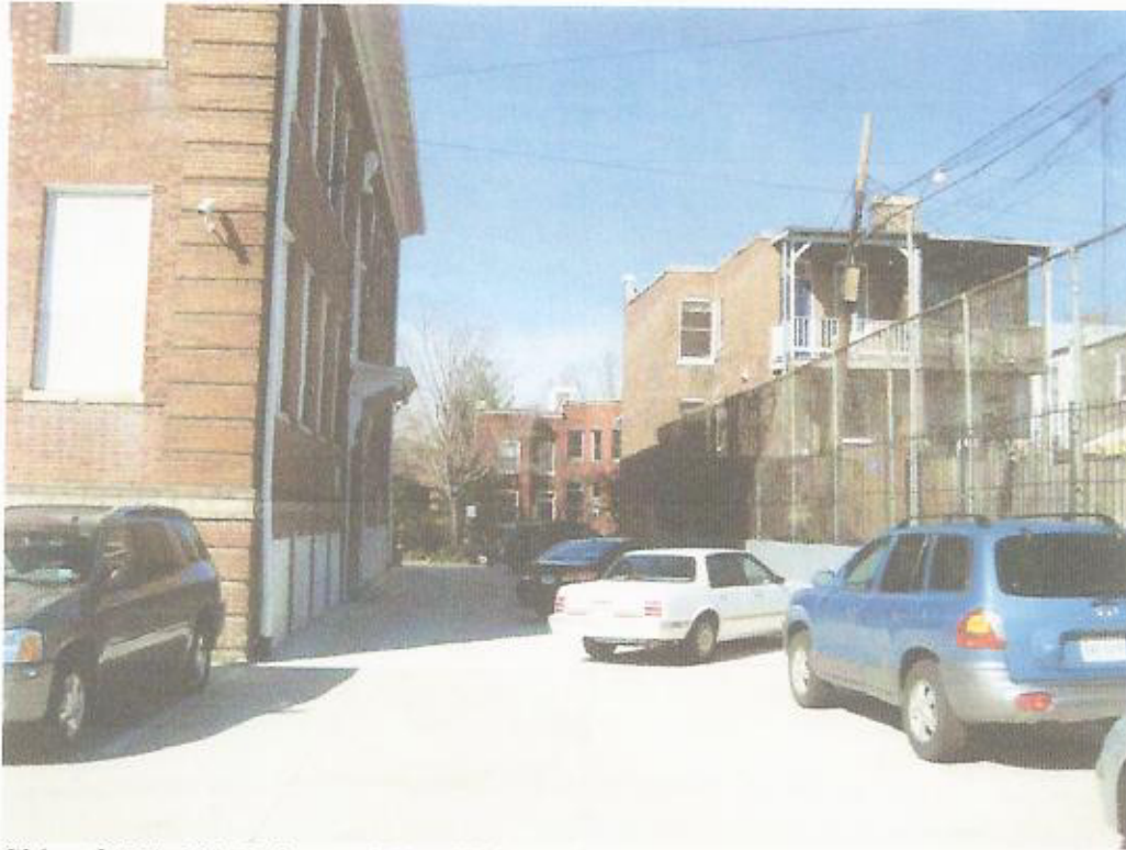
Side of 901-903 D Street, N.E. (Side Parking; Looking towards D Street, N.E.)
