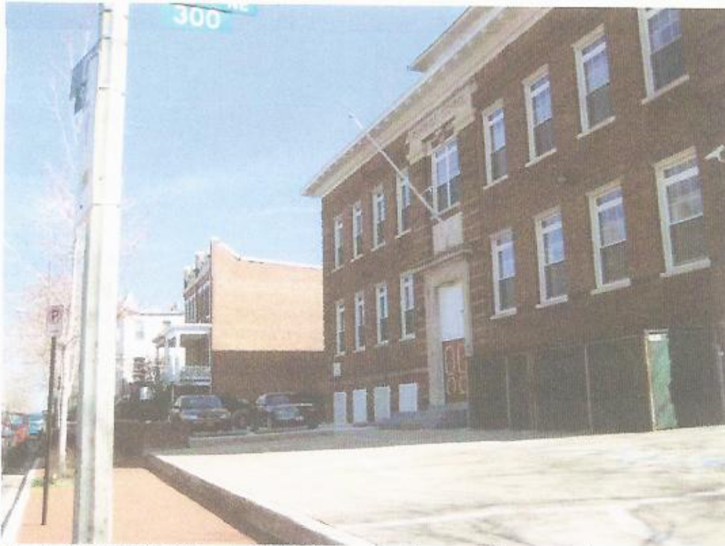
Front of 901-903 D Street, N.E. (Facing the front parking spaces)
