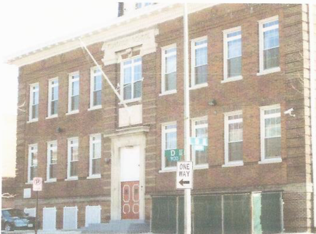
Front of 901-903 D Street, N.E. (Corner of 9 th and D Street N.E.)
