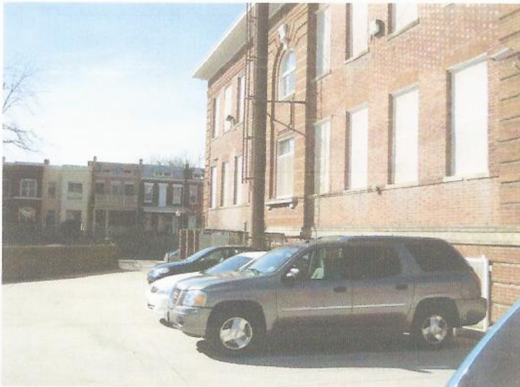
Back of 901-903 D Street, N.E. (Parking Lot)
