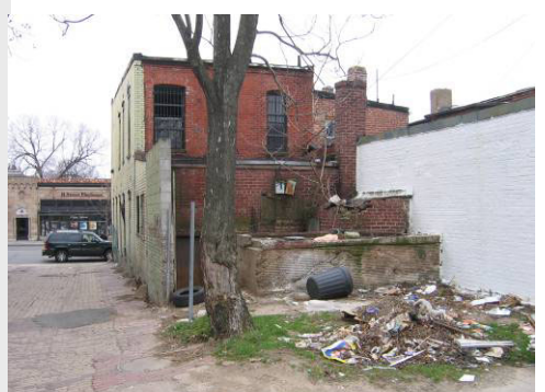
1362 H Street Illegal Dumping – Owner has been fined for not fencing this vacant building
