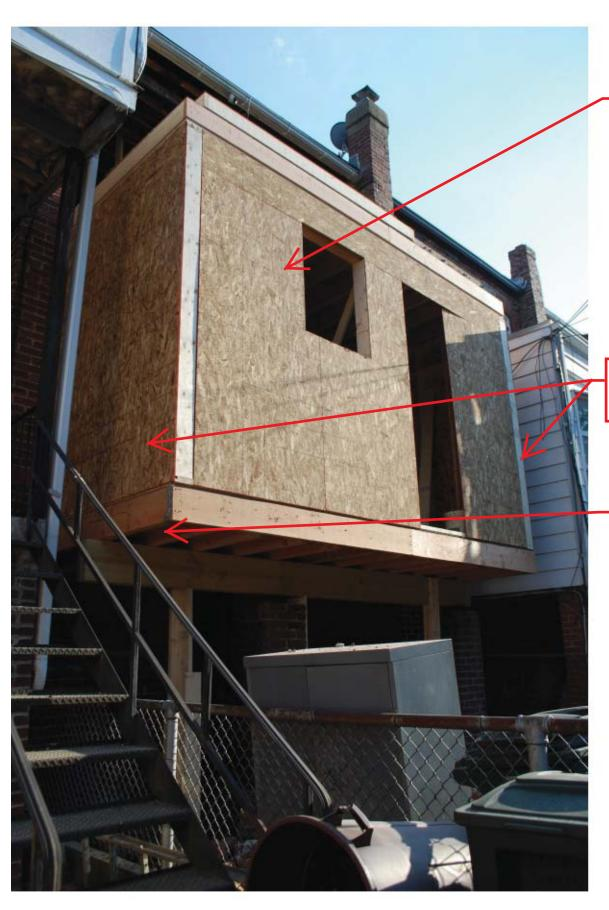
addition was not permitted, exceeds original footprint of porch, boundary survey and wall check were not performed
