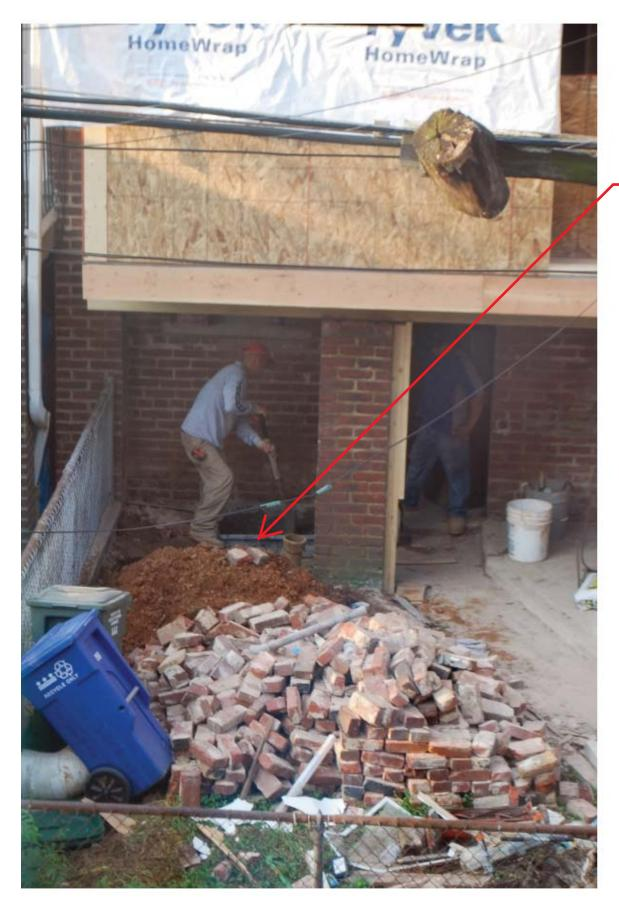
additional footing and pier was constructed (after the addition was in place) without a footing inspection
