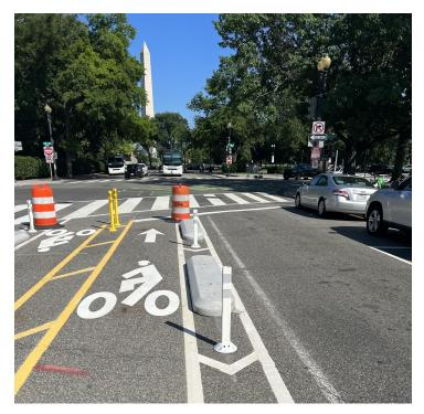
**Travel lane narrowing to reduce vehicle speeds**. The drawings do not provide lane width measurements for either the cycle track or the vehicle travel lane. We request that DDOT endeavor to narrow the vehicle travel lane to 11 or 10 feet to slow vehicle travel and use that additional space to expand the width of the parking bay on the east side and expand the width of the protected bicycle travel lane on the west side.
