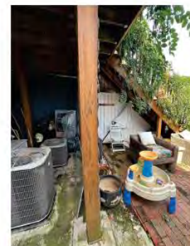
EXISTING STEPS TO GRADE
