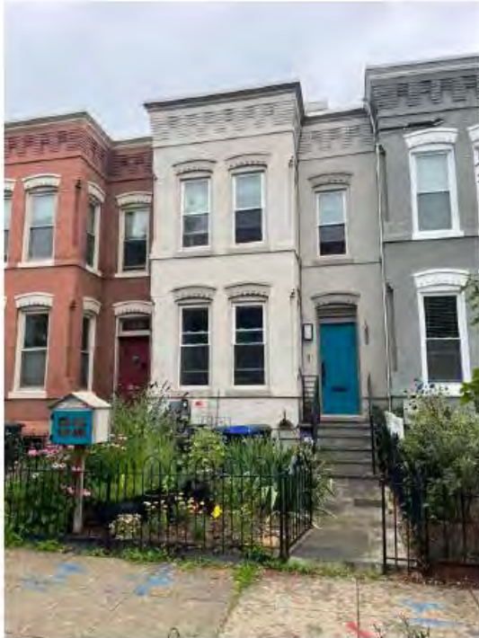
EXISTING FRONT FAÇADE, F STREET NE
