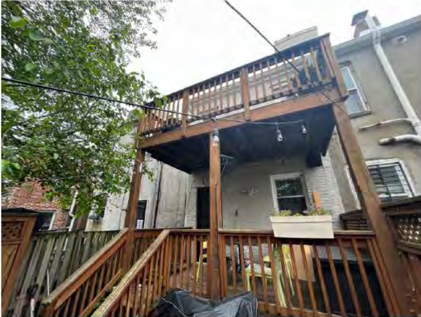
EXISTING COVERED PORCH
