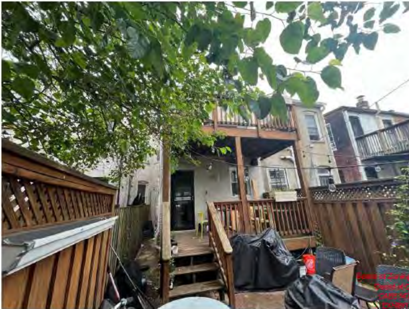
EXISTING REAR FAÇADE
