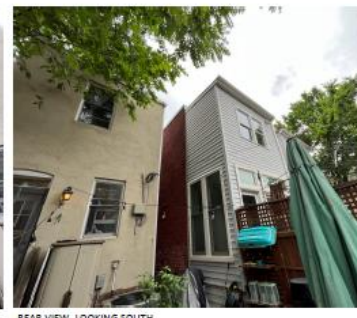
REAR VIEW, LOOKING SOUTH
