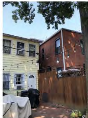
REAR FACADE, LOOKING NORTH
