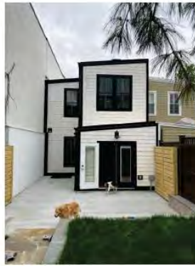
EXISTING REAR FACADE
