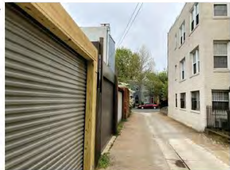
EXISTING ALLEY, LOOKING EAST
