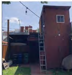
EXISTING CARPORT & SHED(VIEW FROM REAR YARD)
