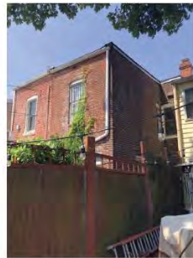
REAR FACADE, LOOKING SOUTH
