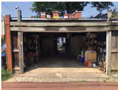
EXISTING COVERED CARPORT(VIEW FROM ALLEY)
