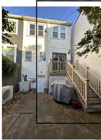
216 11th ST, NE - EXISTING REAR (WEST) FACADE
