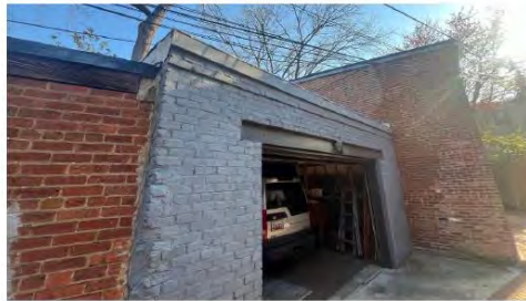
4. VIEW LOOKING NE FROM ALLEY
