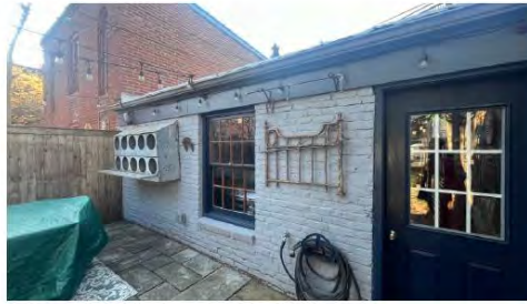
2. VIEW LOOKING S FROM REAR YARD OF 917 CONSTITUTION AVE NE
