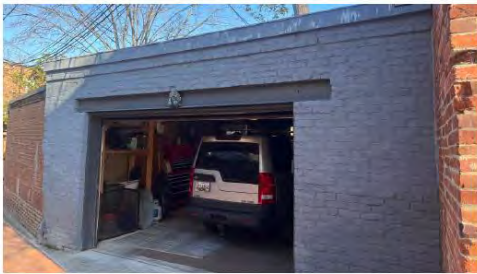
3. VIEW LOOKING NW FROM ALLEY
