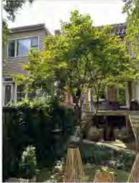
REAR FACADE: LOOKING EASTWARD
