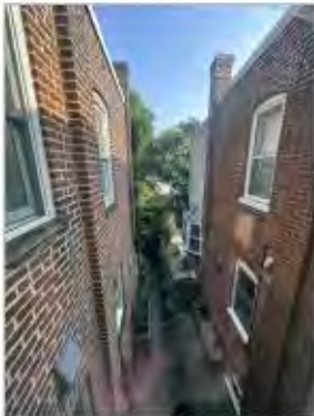
VIEW OF DOGLEG CONDITION FROM SECOND LEVEL
