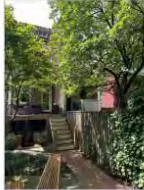
REAR FACADE: LOOKING WESTWARD
