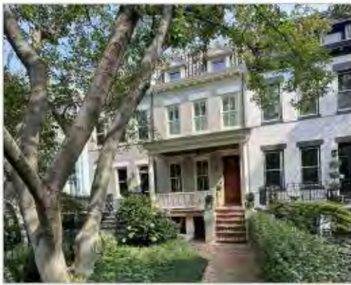
FRONT FACADE: VIEW FROM YARD
