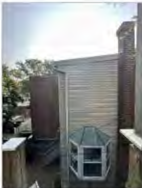
VIEW FROM 2ND LEVEL PORCH LOOKING EAST
