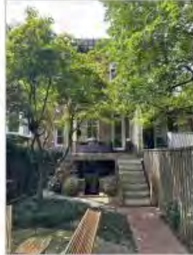
REAR FACADE: VIEW FROM YARD
