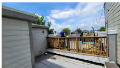
VIEW 5 EXISTING ROOF DECK FROM NEAR STAIR POP UP
