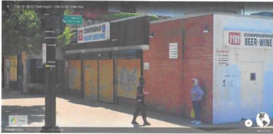
North Elevation of 1101 H Street.
