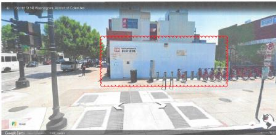
West Elevation 1101 H Street, NE.
