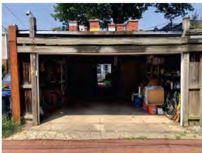
EXISTING COVERED CARPORT(VIEW FROM ALLEY)
