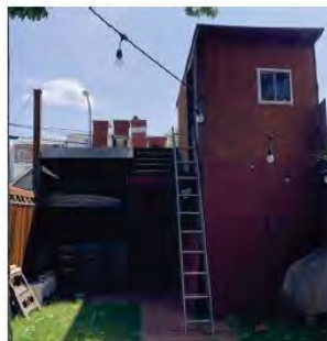
EXISTING CARPORT & SHED(VIEW FROM REAR YARD)
