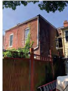
REAR FAÇADE, LOOKING SOUTH
