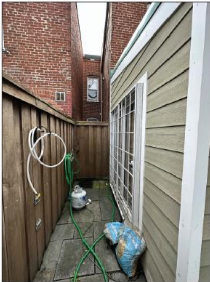
view of dogleg and side of existing 1-story addition
