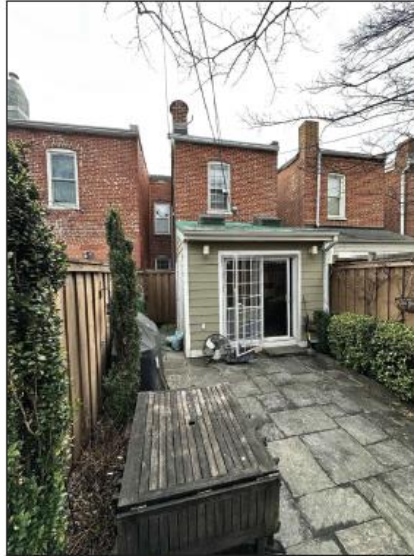
view from rear yard
