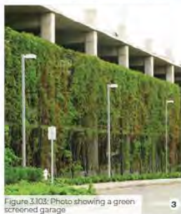
Figure 3.103: Photo showing a green screened garage
