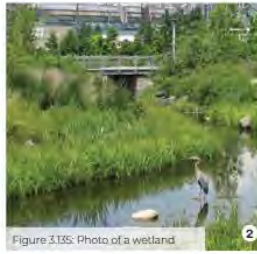
Figure 3.135. Photo of a wetland
