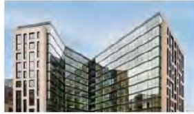
Figure 3.57: The Margate apartments in Washington DC's Union Market District uses a mix of opaque material and glazing to maximize light and views.
