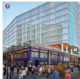
Figure 3.48: Another example at The Wharf in Washington DC illustrates how a terrace can occupy space where building frontage does not meet the streetwall, and allows the terrace to overlook the street and the water.
