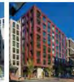
Figure 3.55: Brick and masonry as primary materials and recessed balconies in City Ridge DC.
