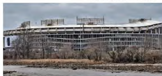
Figure 1.14: Photograph showing RFK Stadium prior to demolition
