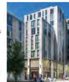
Figure 3.54: Terracotta panels as primary material and vertical orientation at City Center DC.
