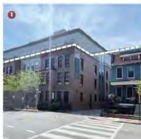
Figure 3.40: This recent multifamily apartment building in Hill East uses a change in material and change in plane (setback) to break down the building's massing and maintain the streetwall height of the existing low-scale rowhouse neighborhood.
