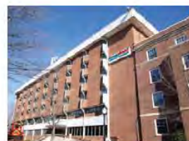
Figure 130: Photograph of BridgePoint Hospital
