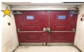
Interior view of side doors south side
