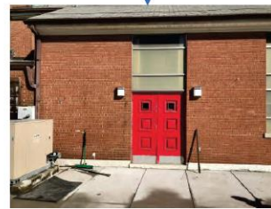
North Carolina Ave – North Side
