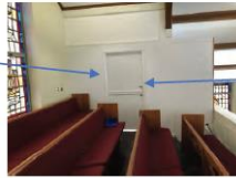
Locked Security Room
