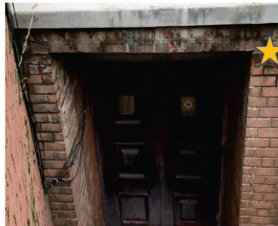
North Carolina Ave - North Side
