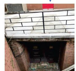
North Carolina Ave – North Side
