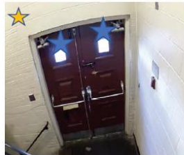
Interior view of side doors north side
