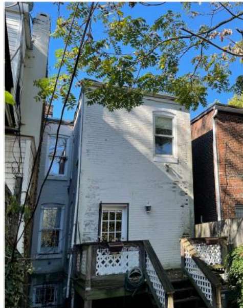
EXISTING REAR FACADE
