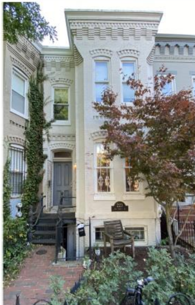
EXISTING FRONT FACADE
