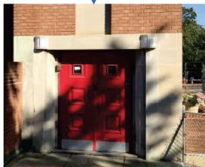
North Carolina Ave – North Side
