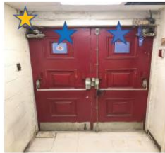
Interior view of side doors south side
