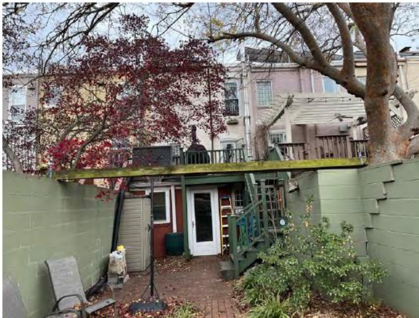
EXISTING REAR FACADE
