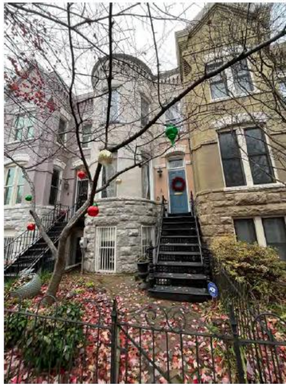
EXISTING FRONT FACADE
