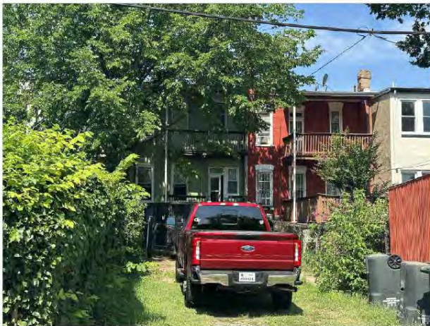
view of rear facade from alley
