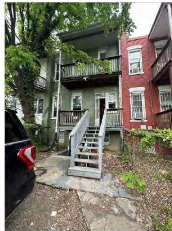
view of rear facade from yard
