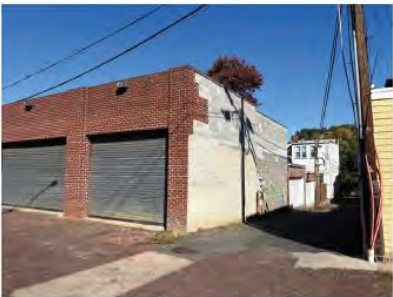
EXISTING GARAGE AT 1223 F STREET NE
