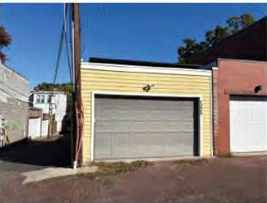
EXISTING GARAGE (SOUTH VIEW)
