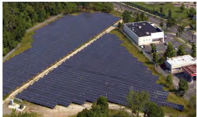
Oxon Run Park, 2.65 MW
