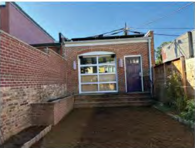
EXISTING GARAGE (NORTH VIEW)
