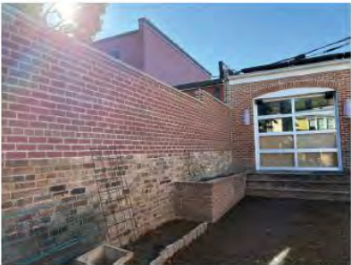
EXISTING GARAGE (NORTHEAST VIEW)
