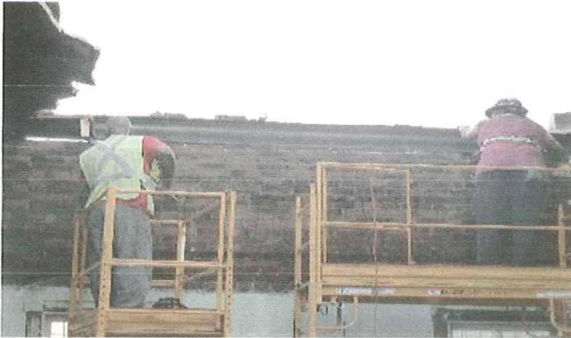
Hand decon of cornice.
