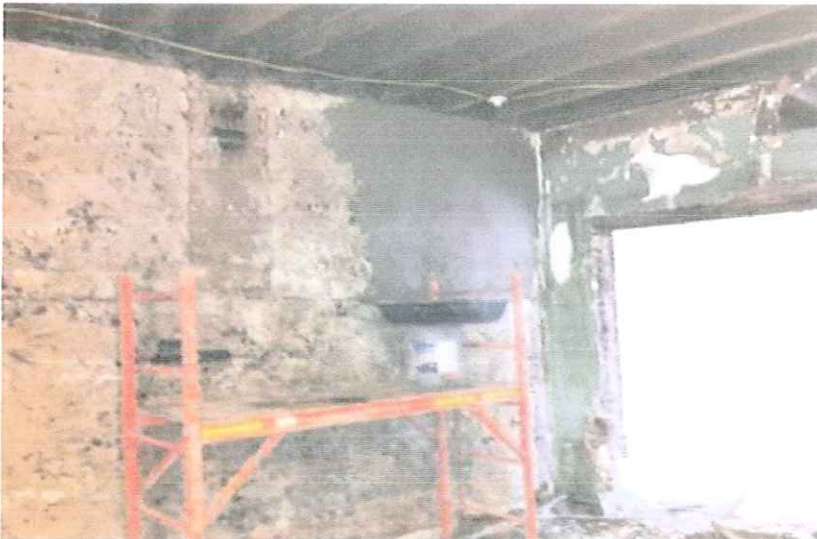
Parging of falling and deteriorating brick and grout.
