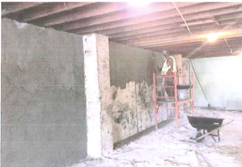
Parging of falling and deteriorating brick and grout.
