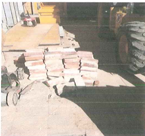
Salvaged brick, coursing review.
