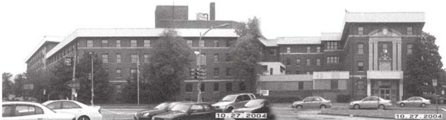
View of Existing South Facade and Southwest Corner
