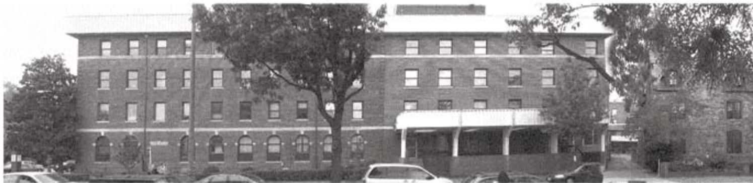
View of Existing East Elevation
