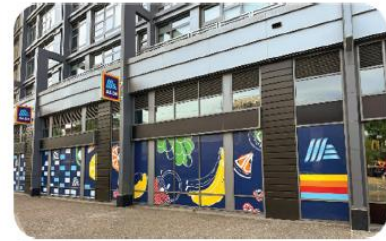
Some storefronts are designed with clear glass, but cover them with graphics, negating storefront visibility requirements.
