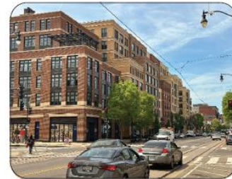
Rec. 21: Photo of building at street level to show pedestrian experience and variety of scale in large, new building.
