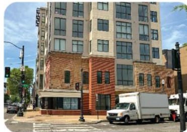
Only one project on H Street (corner of H and 4th St NE) appears to have used the facade preservation bonus.
